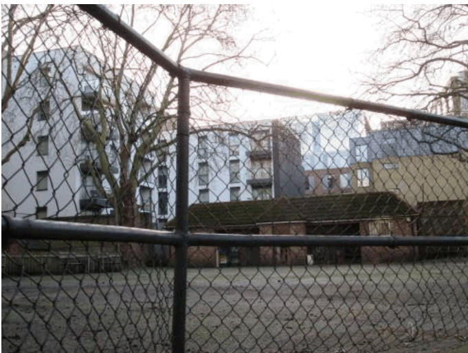
Orchard Building looking south across Seward Street playground
