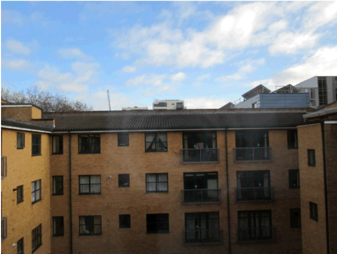
Silverdale Court internal courtyard looking east
