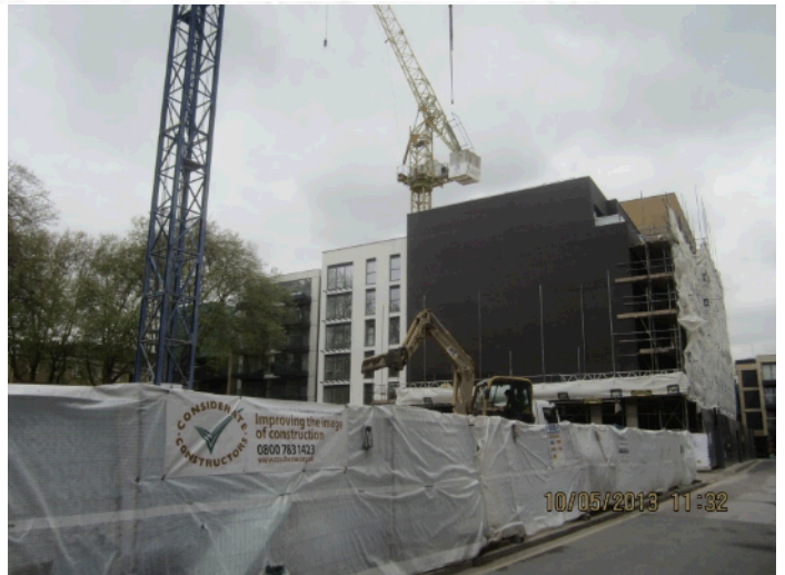
Orchard Building looking east from Pear Tree Street during construction (prior to construction of frontage building)
